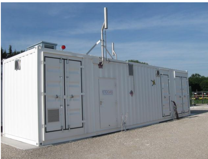
Front wall of the ETOGAS Electrolysis Container
